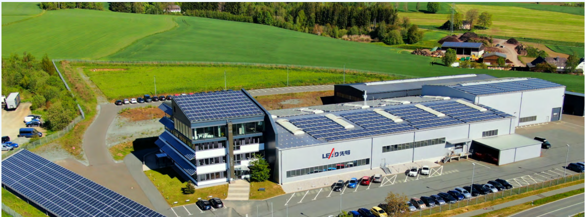
Photovoltaic installation at the Naila factory in Germany
